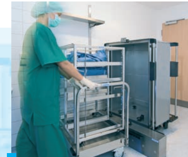
■ Docking at the transition board
